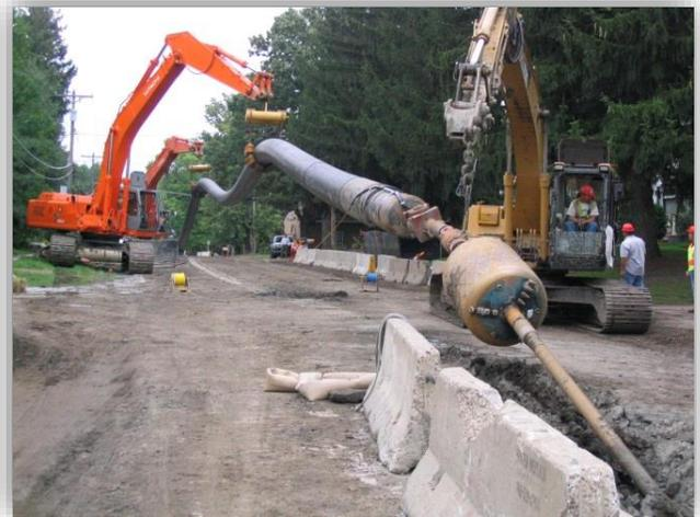
DriscoPlex® HDPE piping is an excellent choice for rehabilitating deteriorated pipelines. Trenchless rehabilitating options include sliplining a smaller HDPE pipe into an existing pipe and pipe bursting, which involves expanding or breaking an existing pipe into the surrounding soil while simultaneously pulling in the new HDPE pipe. See Chapters 11 and 16 of the PPI Handbook of PE pipe for additional information.
